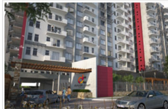
Developed by Costa Zervas Projects, an established developer in Tshwane with extensive experience in residential and commercial developments, the apartments are priced from R595 000 for a studio apartment to R1.665 million for a two bedroom apartment.
